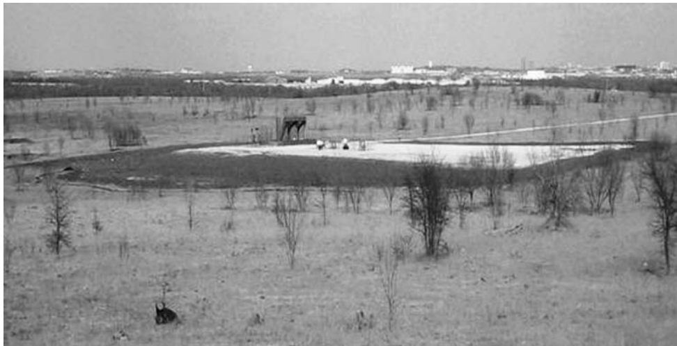
Fig. 2 A typical gas well site consisting of an inner gravel-covered pad and surrounding disturbed area. A mulch filter berm, required by city ordinance and designed to prevent runoff, can be seen at the edge of the disturbed area
